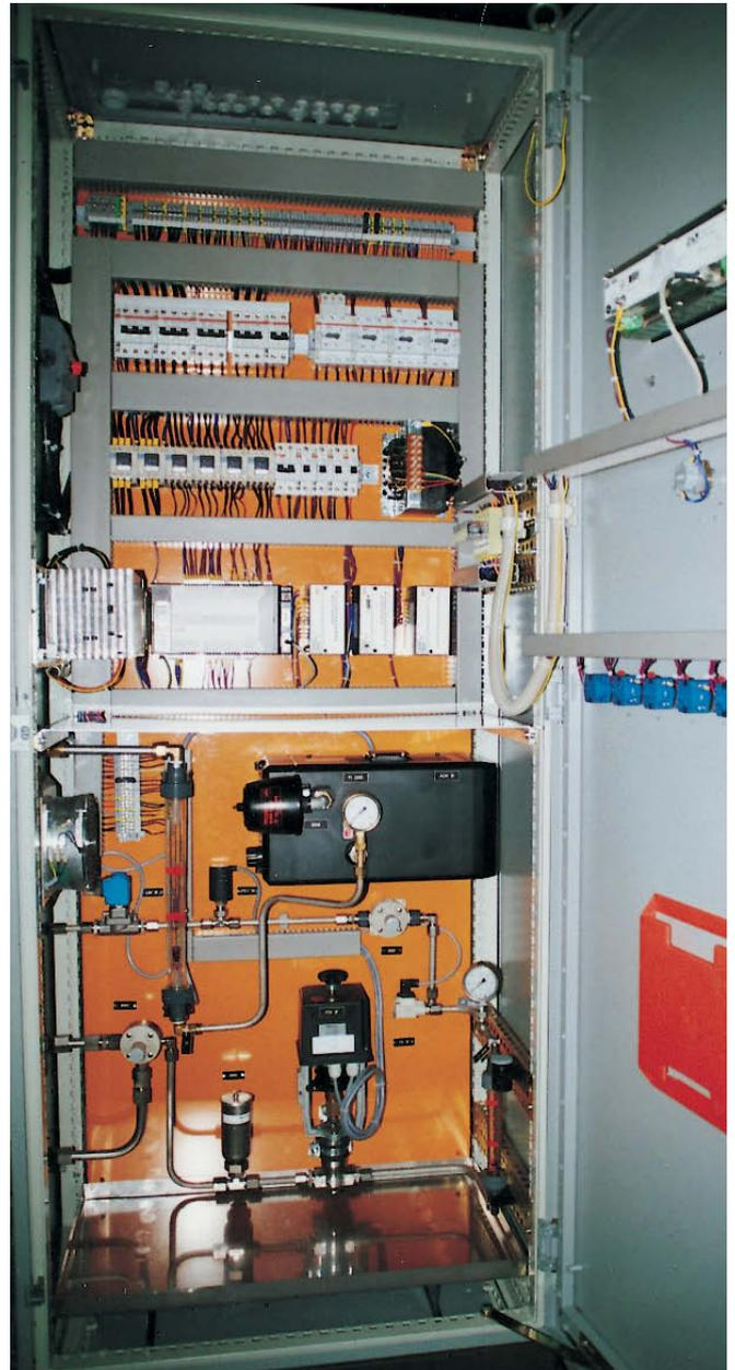
Control panel with PLC system and dosing unit
