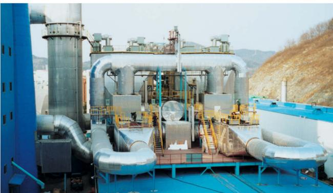
Dual-DeNO<sub>x</sub> catalyzer unit for glass smelters 304,600 m<sup>3</sup>/h
