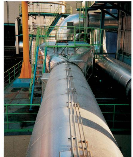
DeNox catalyzer unit for gas-fired glass smelting process
