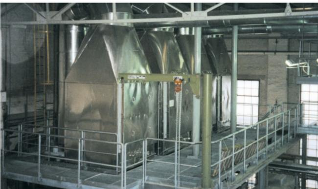
2 Dual-DeNO<sub>x</sub> catalyzer units for heavy oil fired boiler, 56,000 Am<sup>3</sup>/h each
